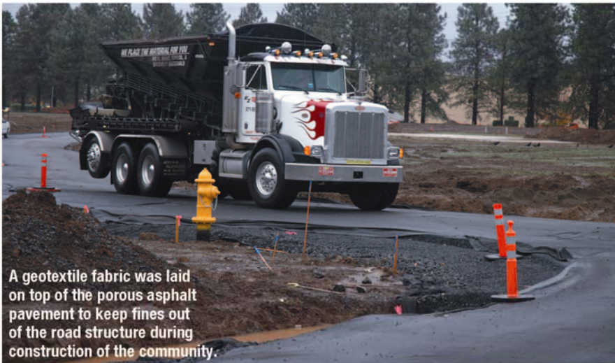
The crew from North Santiam Paving lays the 2-inch pervious wearing course for the pavement.
