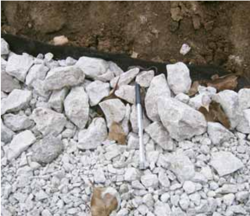
Coarse stone and "choaker" aggregate used for stone recharge bed.
