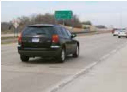
I-435 in Kansas was a concrete pavement in need of rehabilitation.
