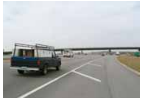
The new HMA overlay provided a much smoother and quieter alternative.
