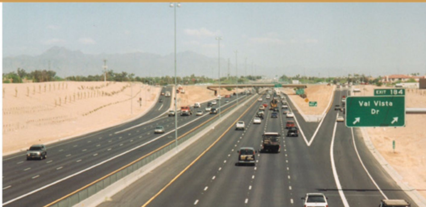
The asphalt rubber overlay on Superstition Freeway (US 60) prompted numerous compliments from neighbors.
