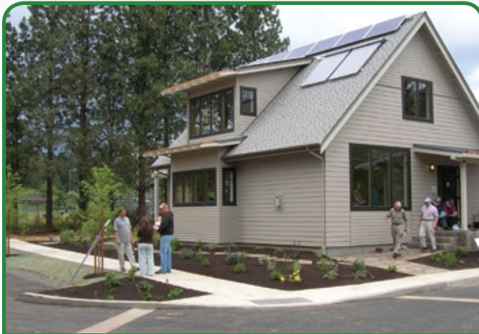
POROUS ASPHALT STREET IN FRONT OF A LEED PLATINUM MODEL HOME
